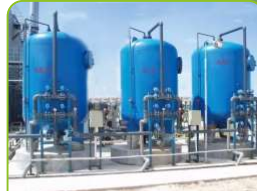
REVERSE OSMOSIS SYSTEM , SOFTNER , D M PLANT
